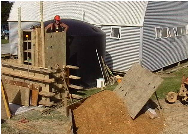
Figure 12: First rammed earth wall corner section
