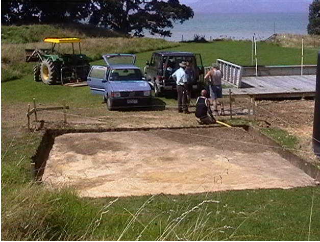
Figure 13: Dewatering perimeter foundation trench
