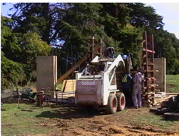
Figure 22: Placing mixture into formwork
