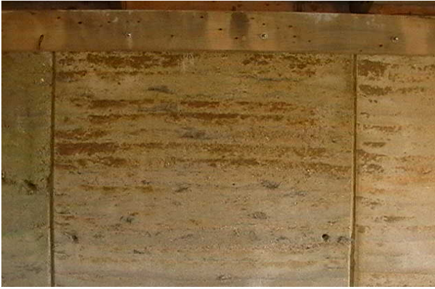
Figure 15: Fibre-reinforced earth wall panel
