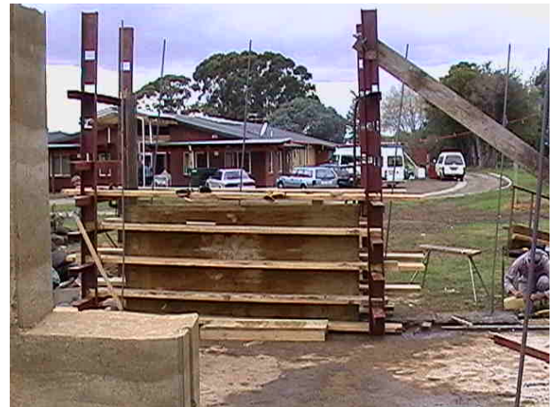
Figure 20: Modular false-work and formwork
