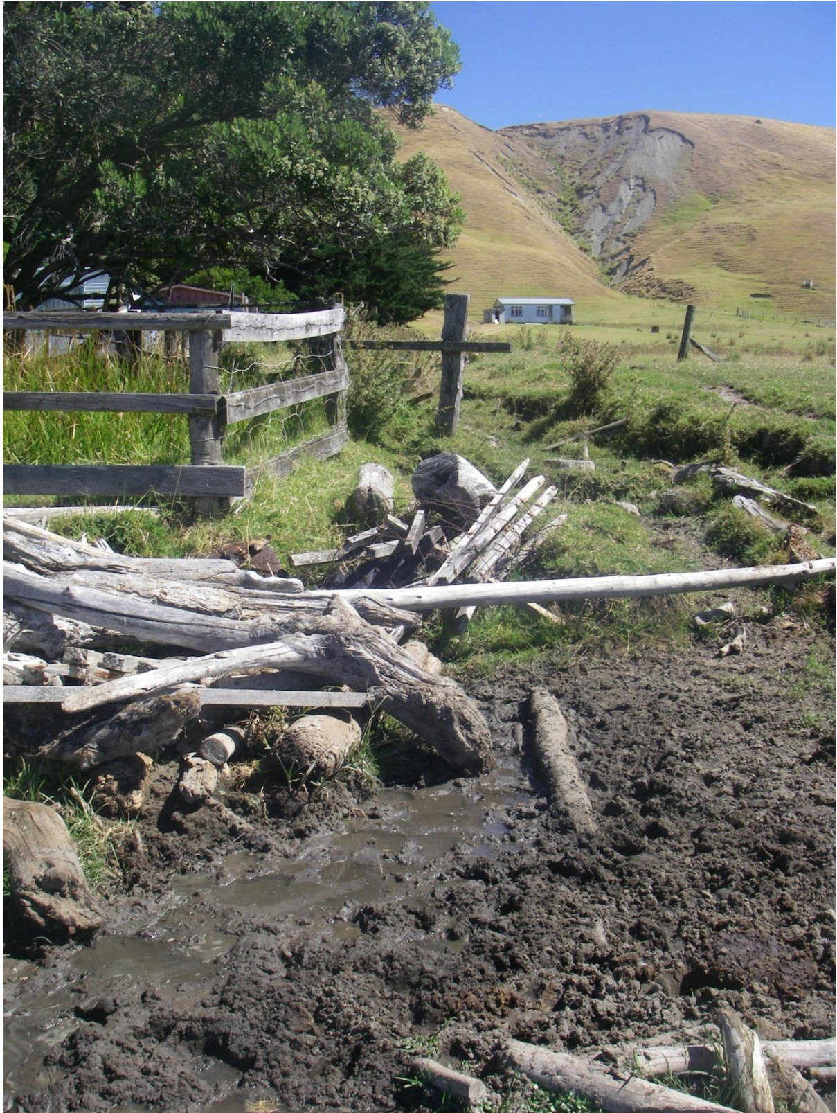
Figure 5: Stream outlet in foreground and stream hillslope erosion in background.
